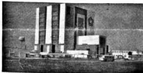
The awesome VAB at the Kennedy Space Center. How could a rocketeer go to Florida and not visit KSC?
